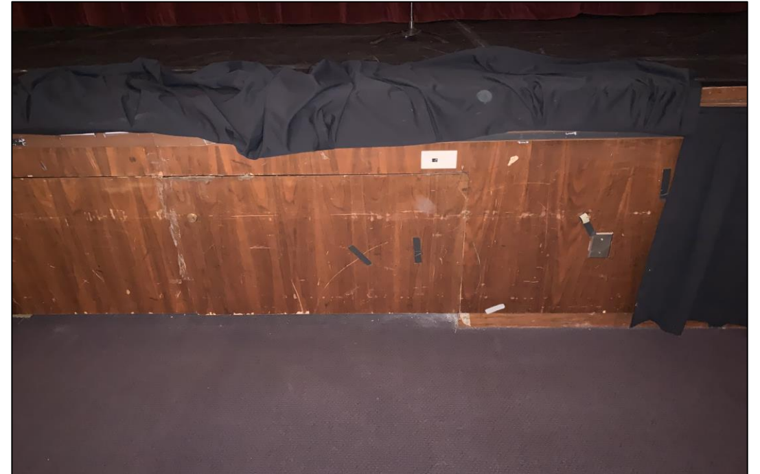
Auditorium Stage Front Finishes
